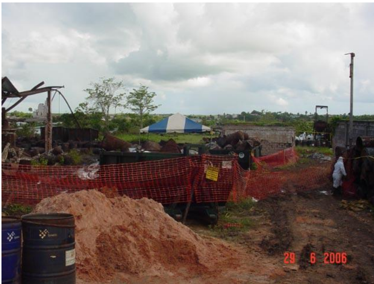
❖ Isolation and demarcation of Site
